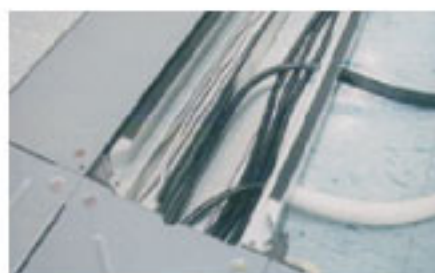
Using cross and straight separator power lines and data lines can be separated.
